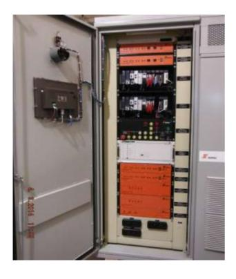
The three equipments installed in Aguacapa of SEPAC brand, belong to the model RAV 1111 2P 440K/250. They are manufactured in Mexico by SERPRO and contain the latest technology of similar excitation systems equipments found in the market.
