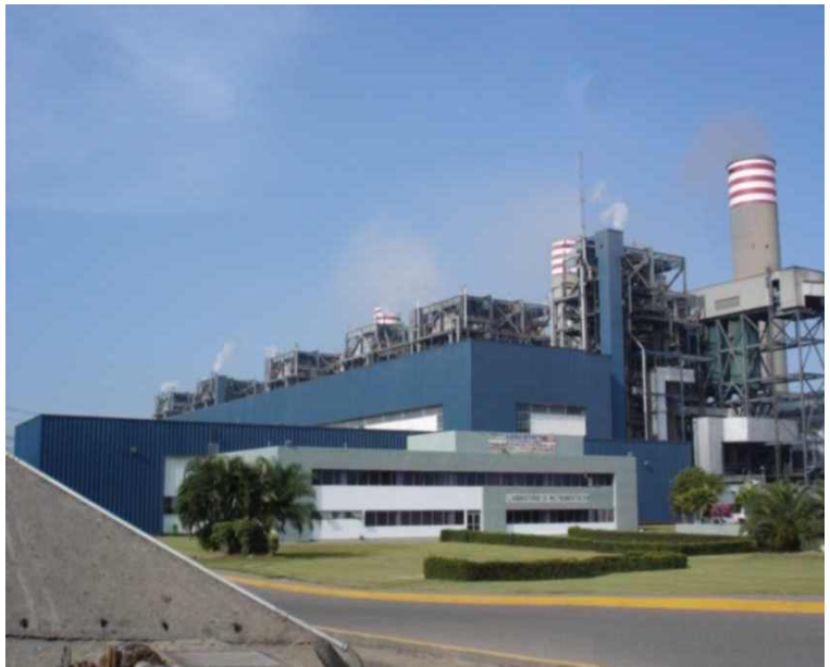
Petacalco thermoelectric plant, one of the most important power plant in CFE. Mexico
